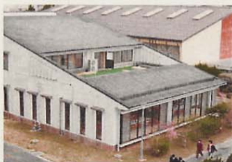
福利厚生施設 Welfare Facilities
